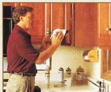
Cabinet Refurbishing - cleaning, degreasing, repairing and polishing
