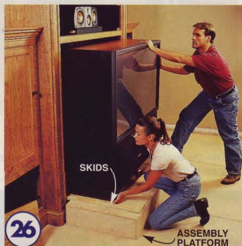
26 Roll the TV home. Here's where your construction platform earns its keep a second time. The 3/4-in. skids bridge your platform to the TV base so you can roll the behemoth into the cabinet without damaging the cabinet, the TV or yourself!
