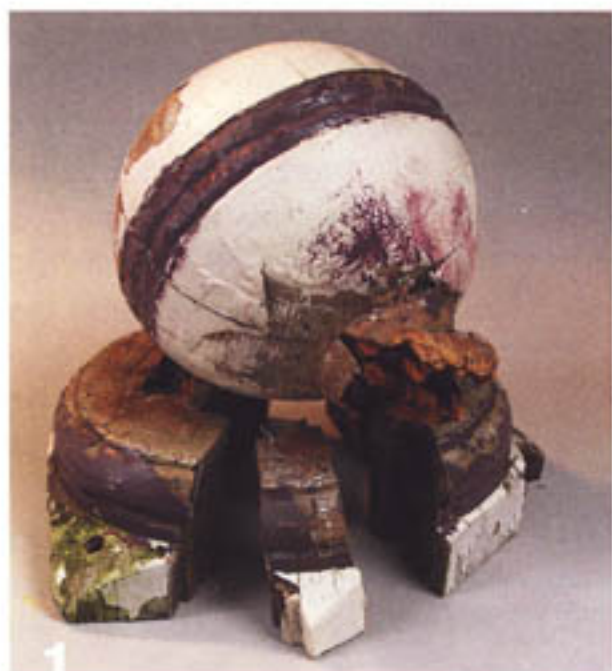
Original newel post cap, rotted.
