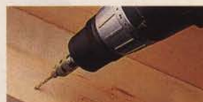
Drill pilot holes
