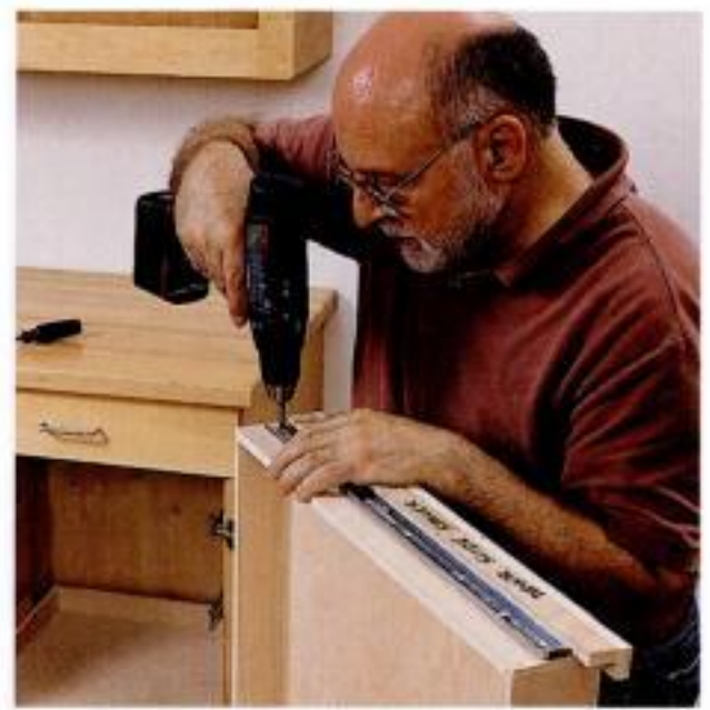
Attaching the drawer slides. Shop-made spacers help align drawer slides during installation.
