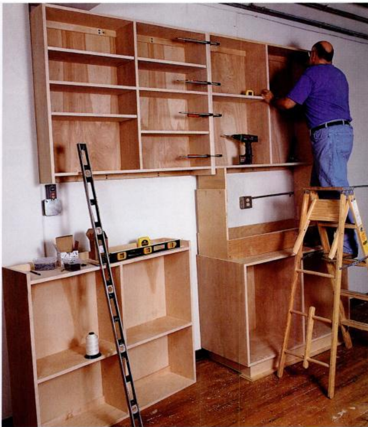
Installing cabinets. Use a crutch to support a wall cabinet while you screw it to the wall studs and to any adjacent cabinet.
