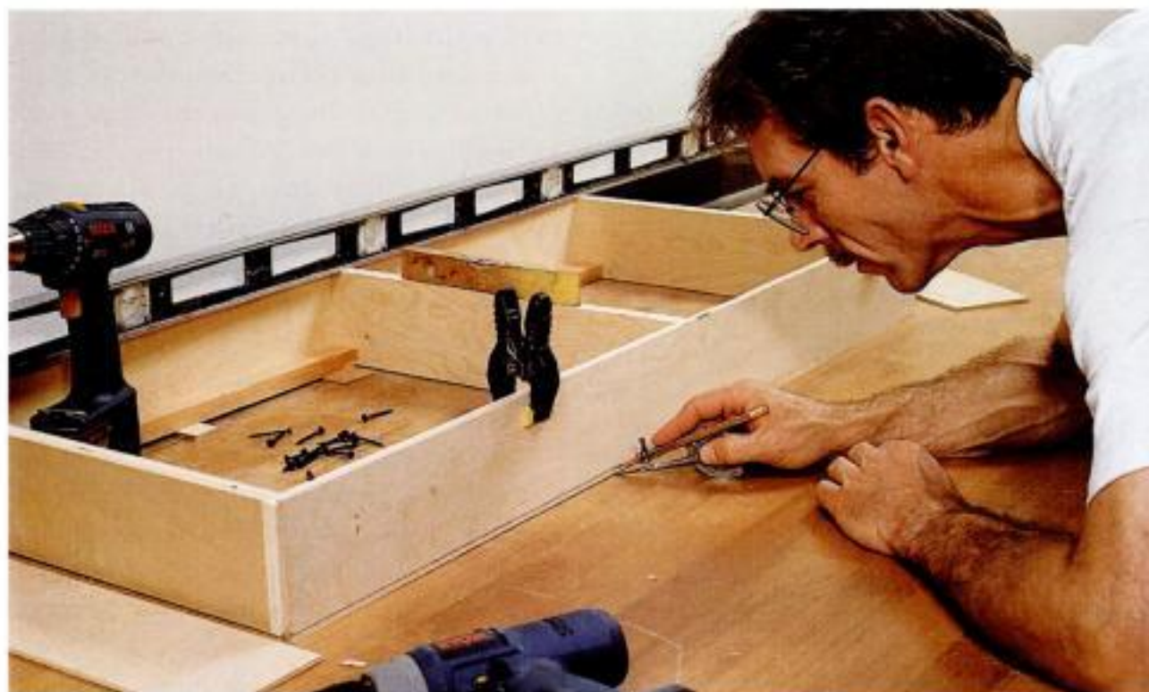
Install the base. After shimming the base level and screwing it to the floor, scribe and attach 1/4-in.-thick facing to the exposed faces of the base.
