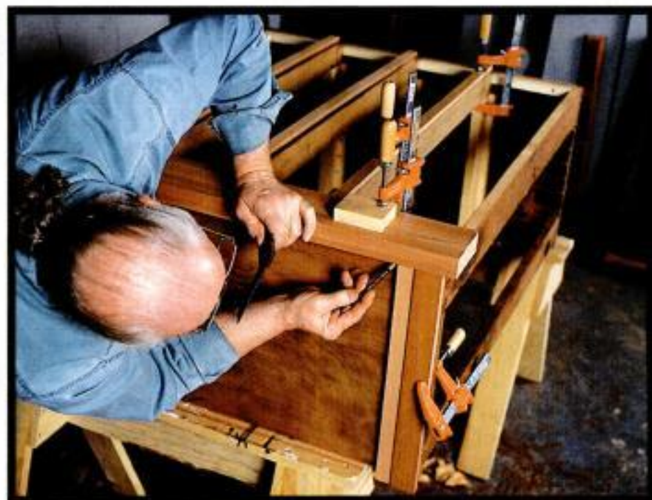
Corner posts and base trim. New, larger corner posts, simple base trim, and matching rail edging give the remade piece a more contemporary appearance.
