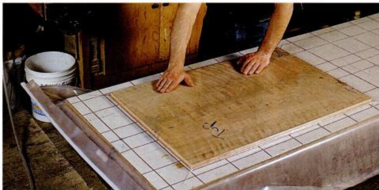
Press the veneer. A vacuum bag and pump system clamps the veneer to the panel. Saporito uses 1/8-in. hardboard cauls over and under the panel to keep the veneer flat on the MDF.
