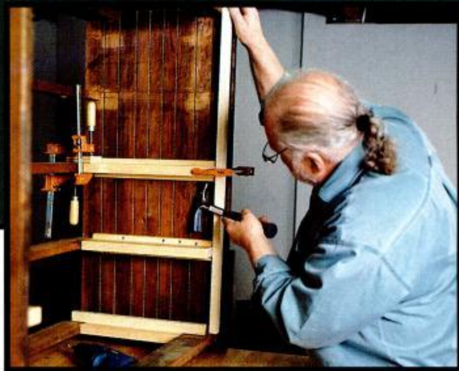
New drawer supports. Installing the T-shaped supports pulls the sides flat. The supports are aligned with front rails and with layout marks on a measuring rod.
