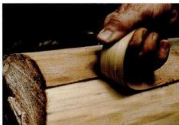
Peel off the strips. Start at one end of the log, and peel off full-length strips one at a time.
