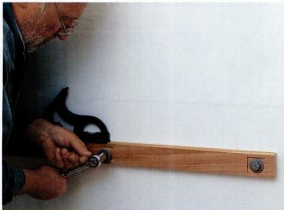
Lagging the ledger. Pockets chiseled in the ledger increase screw penetration into wall studs. Washers help to distribute the screws' holding power.
