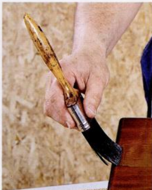
Lift off. When you come to the end of the stroke, lift the brush off the wood while you're still moving the brush forward.
