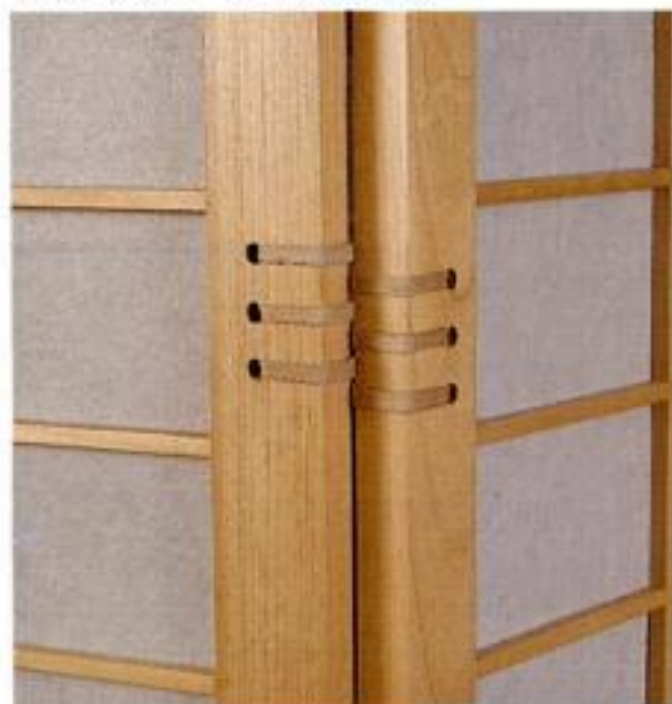
Swing on a string. Ordinary shoelace runs through a series of holes, allowing adjacent stiles to pivot 360°.
