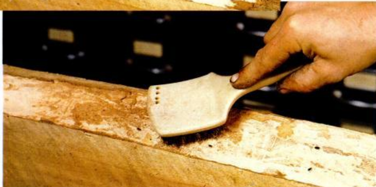
Brush it off. Remove loose debris with a brass brush to avoid harming the surface.
