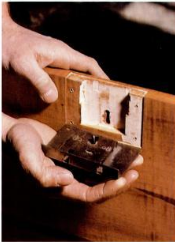
Mortising the lock. The lock fits into a two-tiered mortise. First, mortise for the body of the lock; then carefully mortise for the back plate.
