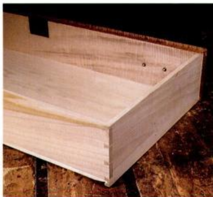
Wrong-way tails. John Wheeler Geer, the original craftsman, cut the tails on the backs of drawers instead of the sides—perhaps as a maker's mark.
