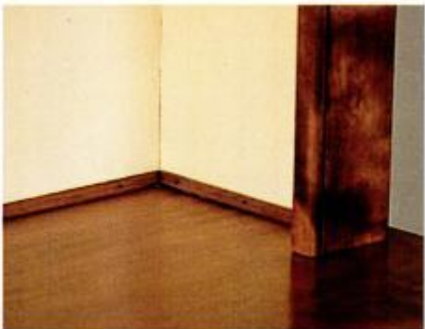
Simple alignment. A mitered cove molding nailed to the countertop registers the upper case.
