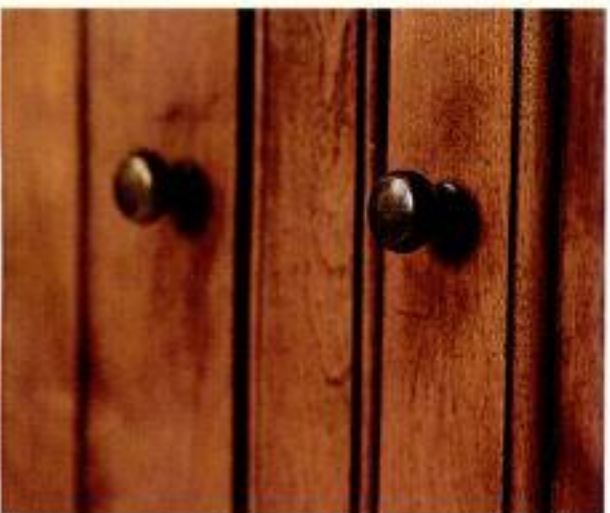
Beads and thumbnails. The thumbnail on the inside edge of the door frame complements the beaded face frame.
