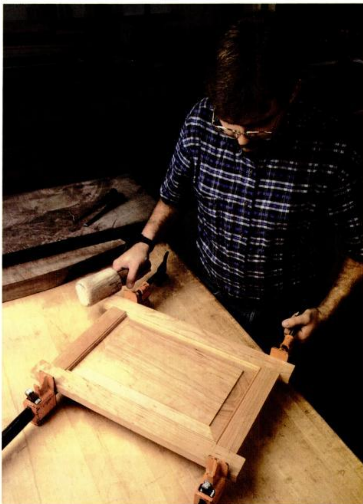
Clamping up. A pair of pipe clamps pulls stiles and rails together around a raised panel. Excess "ears" on stile ends will be trimmed after the glue dries.
