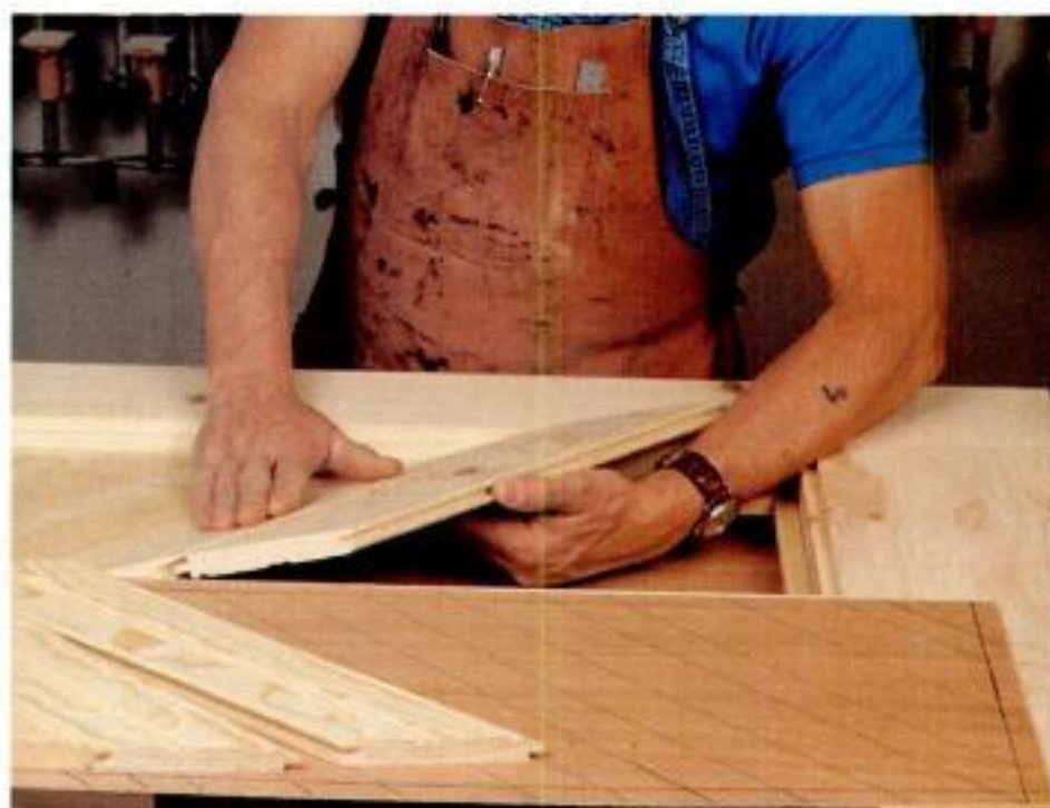
Diagonal paneling. With their ends cut at 45°, T&G boards are fit together to fill the frame opening. Diagonal guide-lines on the plywood panel in the foreground make it easy to lay out the boards.
