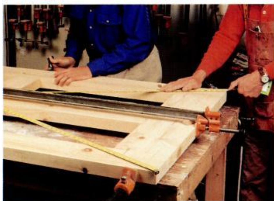
Framed up. The authors clamp up the door, using a pair of tape measures to check for square by comparing diagonal measurements.
