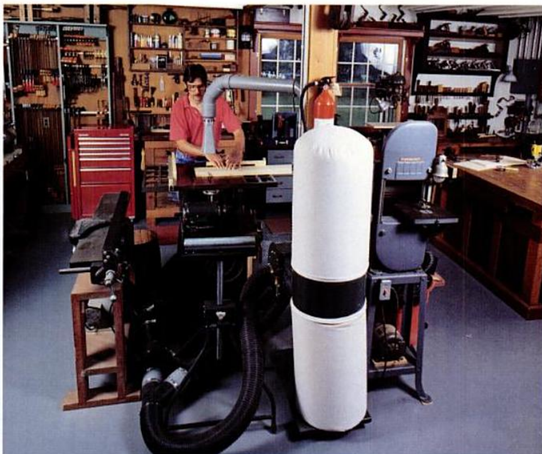
Keeping it clean. Sawdust and chips stay off the floor and out of the air, thanks to this centrally located single-stage dust collector.
