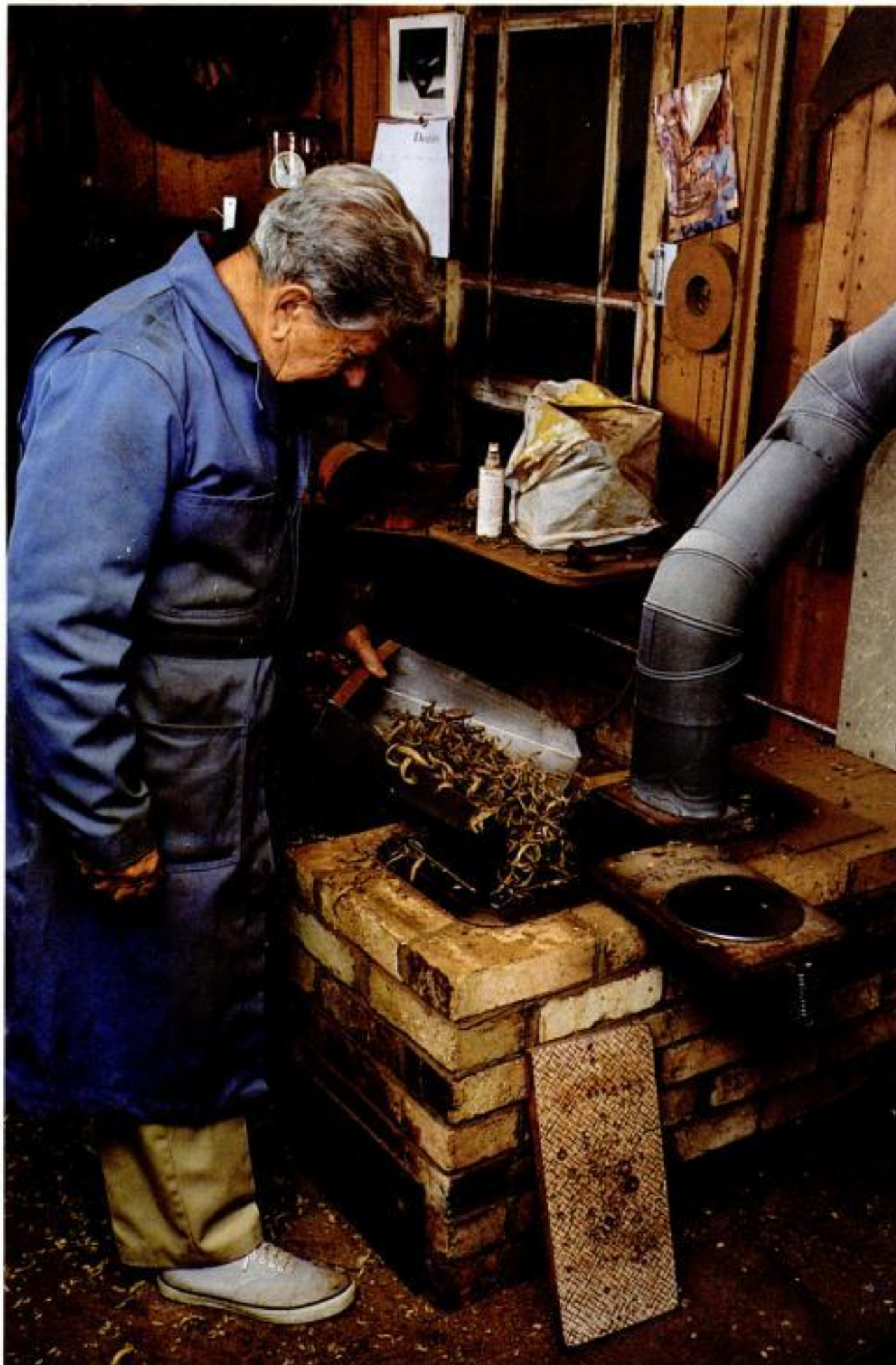
A woodworker's best friend. Woodstoves work double-duty, heating your shop and helping to keep it clean.
