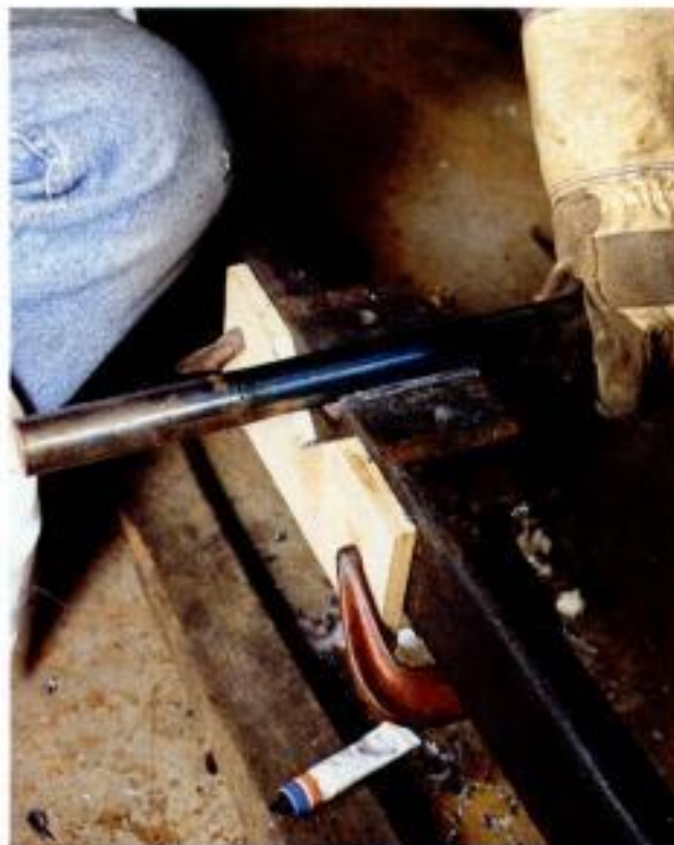
Finding the high spots. A thin coat of Prussian blue dye on the shaft will show where the bearing needs to be scraped to maximize surface contact with the shaft.
