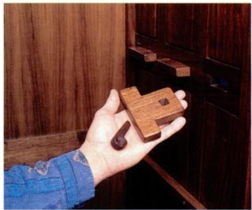
Shelf support option. Tusk-tenoned shelf brackets may be used to support a removable shelf.
