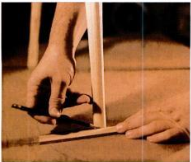
Tracing the feet. Marian marks the compound angle on the legs with a pencil and some scrap.
