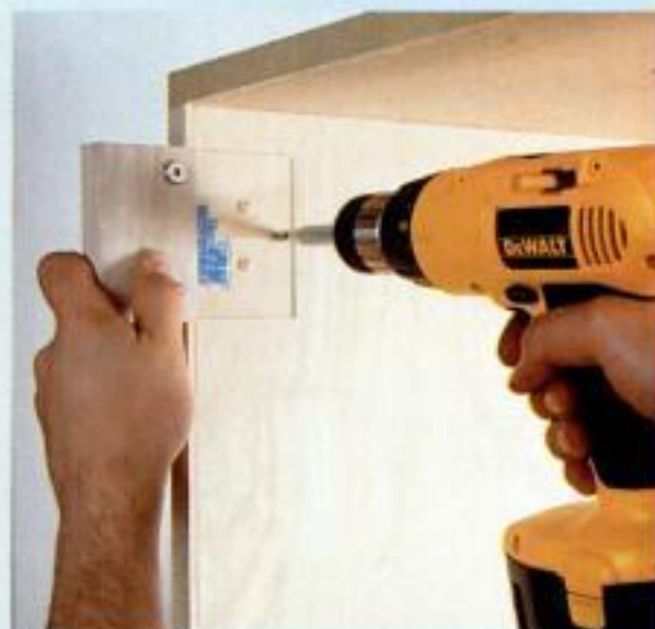
Drilling for the baseplate. Held against the front edge of the cabinet, this jig locates the pilot holes for installing the baseplate.
