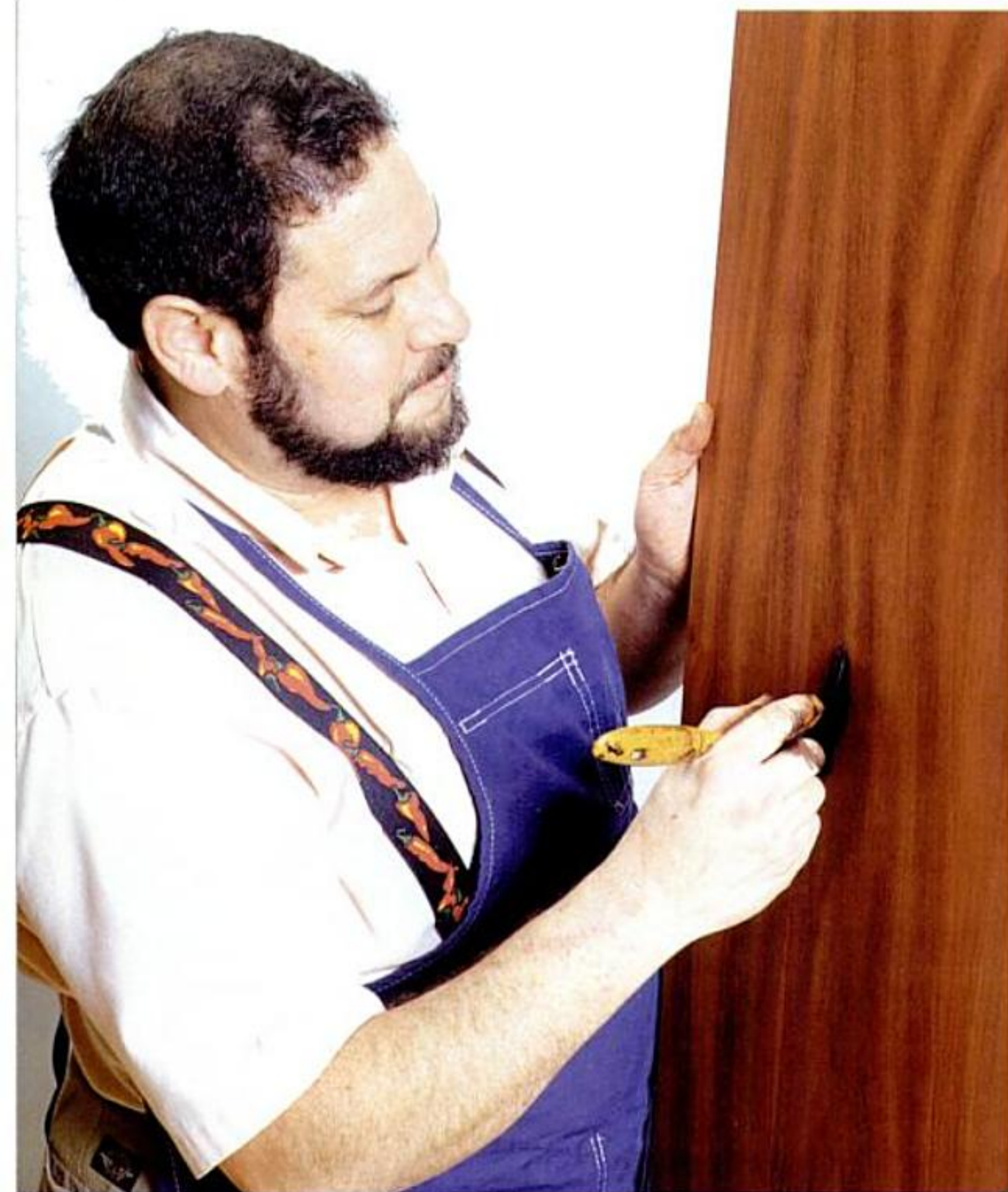
The techniques of ground staining, pore filling, dry brushing (shown here) and wet glazing can add character to your finishes.
