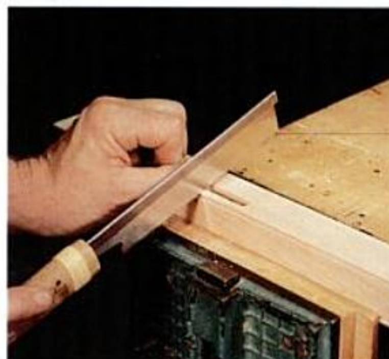
STEP 2: Cut inside your marks to the bottom of the bead with a backsaw.
