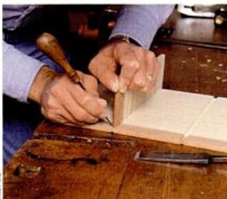
Author marks end of divider by placing it into the dado and using an awl to scribe the cut.
