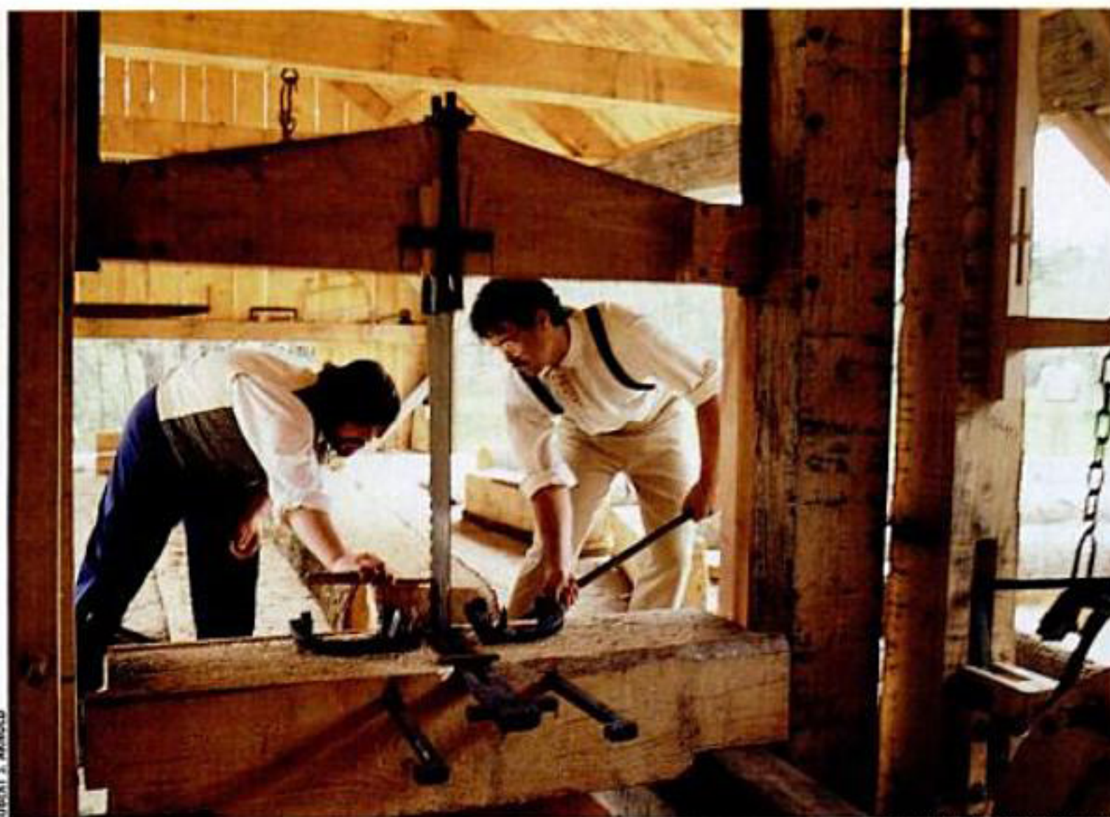
Bringing history to life, two Old Sturbridge Village sawyers prepare a log for the next pass through a re-created 1830s waterpowered up-and-down saw.
