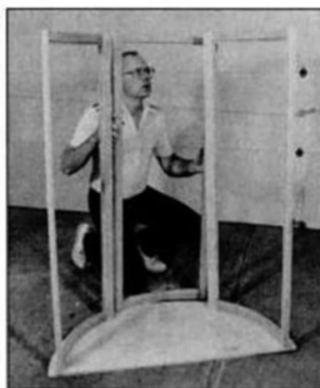
When the frames are completed, position them on a scrap plywood bottom to determine the shape of the cabinet's curve. Use the plywood as a template for the real top and bottom.
