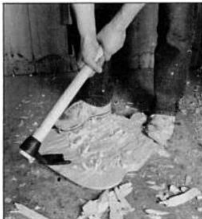
Rough out the dished saddle area on the top of the seat with a gutter adze. Finish the saddle shaping with a scorp (curved drawknife) and travisher (curved spokeshave).
