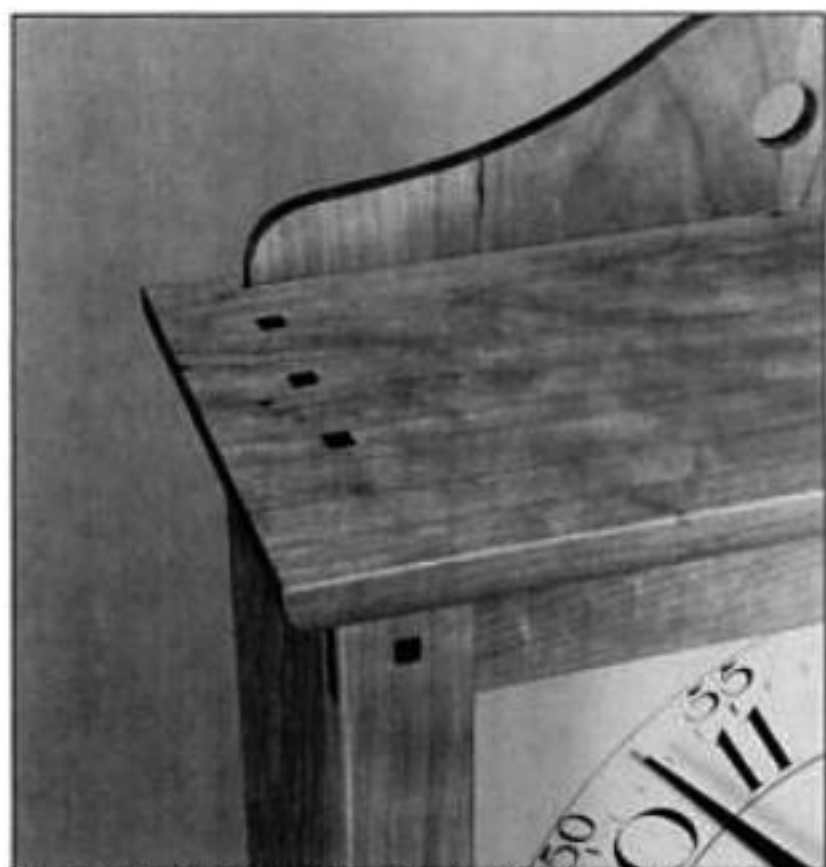
Square-headed dowels reinforce the clock's corner joints and give a traditional appearance.
