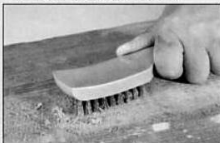
Scrub out any paint or stain that remains in the wood pores with a soft brass-wire bristle brush. Scrub with the grain of the wood.
