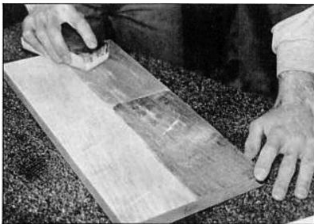
Sanding is the key to a perfect finish. Sand the sealer coat with 220-grit no-fill paper wrapped around a felt block or a blackboard eraser. Here, Camp sands a sample board on which he's applied finish over several different stains.
