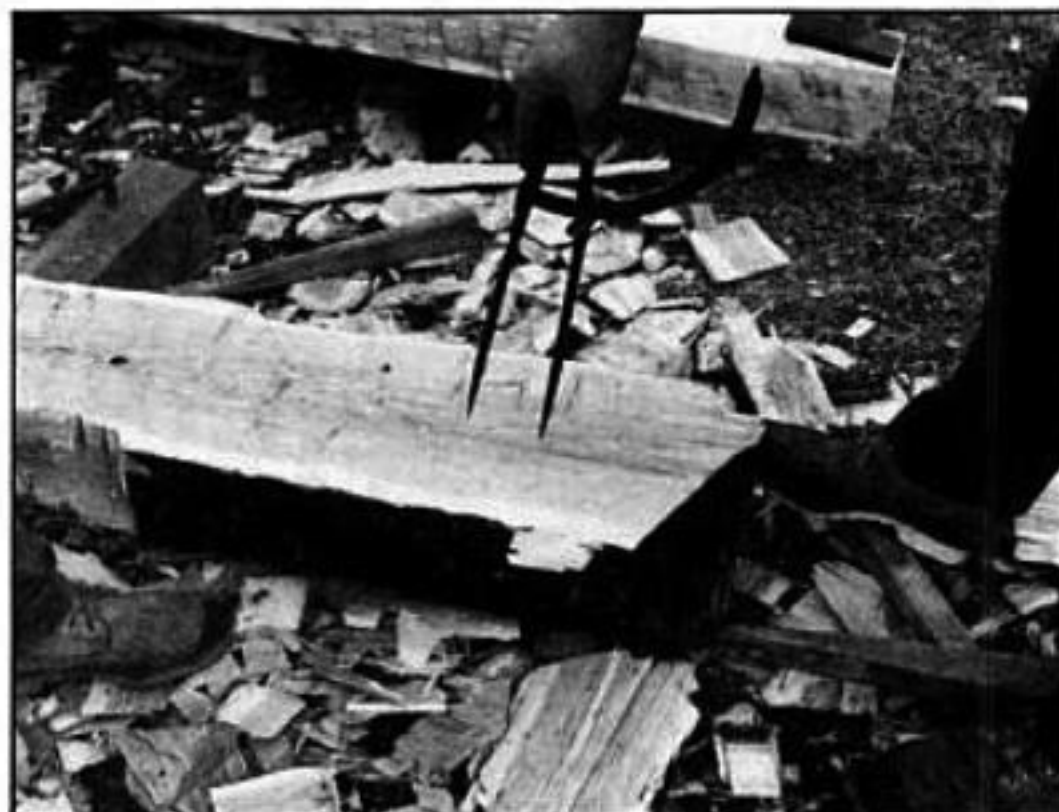
With a large pair of dividers, mark a circle at each end of the log to determine the width of the beam. Snap a chalk line tangent to each side of the circles to mark a boundary line.
