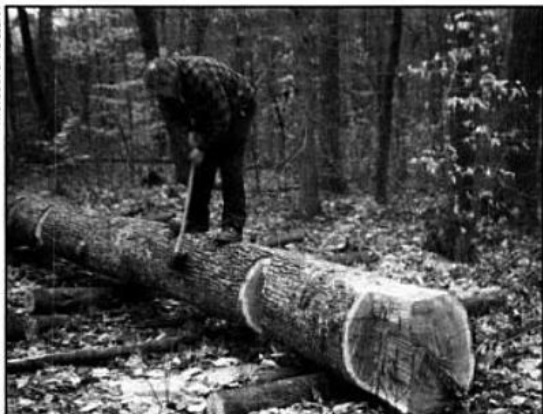
Barn restorer Richard Babcock scores the face of a 20-in. dia. red oak log that will replace the rotted sill of a 17th-century barn in Woodbury, Connecticut.
