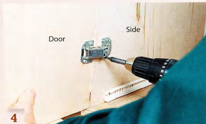
4 Hang the back doors with surface-mount hinges. Screw the hinges to the doors first, then screw the doors to the box.
