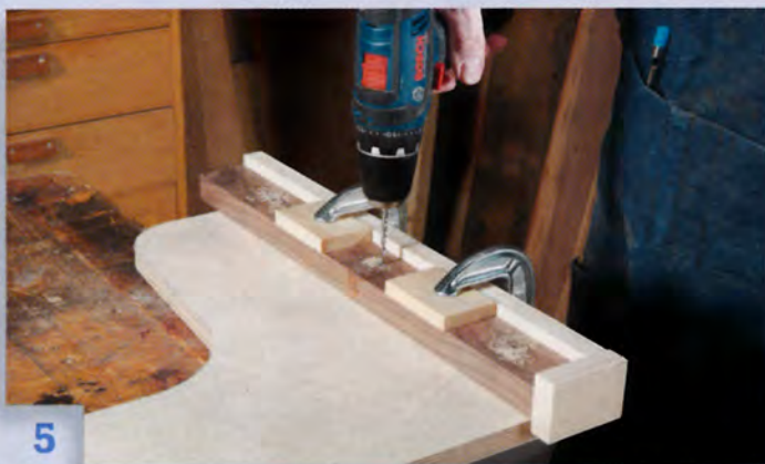
5 Drill holes for the screws that will hold the table together. Using this jig ensures that the holes will be plumb and in the right spot.
