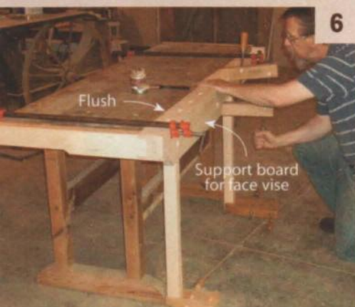
6 Install the fixed jaw with glue and lag bolts, making sure it's flush with the existing bench top. The board glued on the bottom of the fixed jaw supports the Federal-style double-screw face vise.
