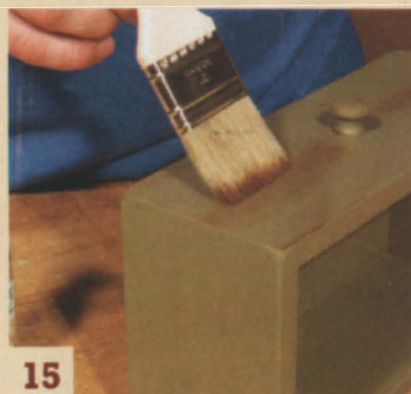
15 Add brown glaze to imitate wear and handling.
