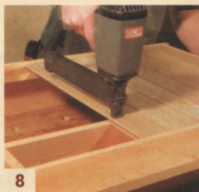
8 Attach the back boards, which are thin pieces of tongue-and-groove paneling.
