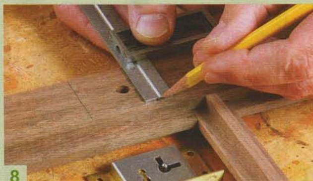
8 Transfer both measurements to the inside face of the door.
