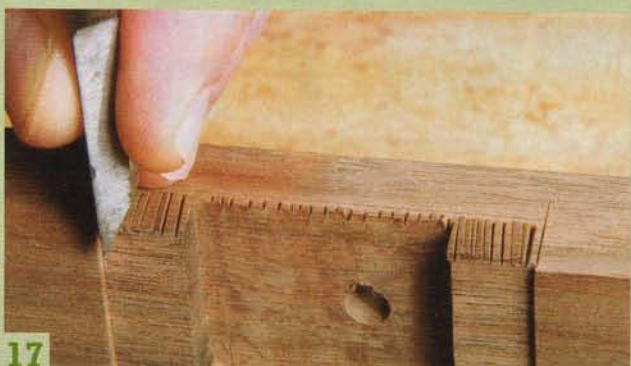
16 Place the lock back into the mortise. Scribe around the three sides of the back plate's edge.
