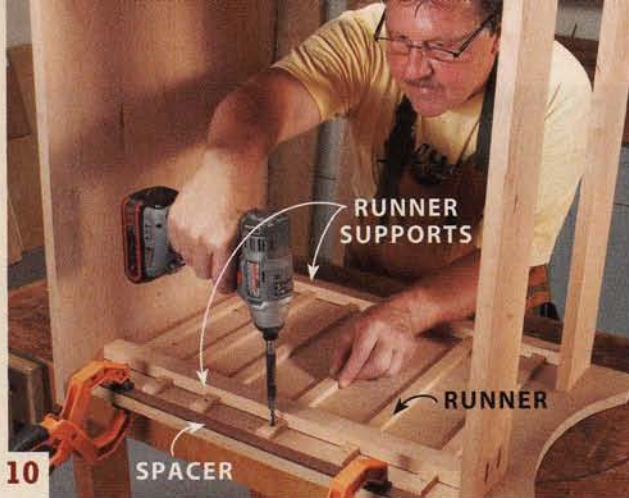
10 Use supports and a spacer to accurately position the drawer runners for fastening. Make the supports by cutting dadoes in a wide board and then ripping it. The spacer establishes the drawers' setback at the front.
