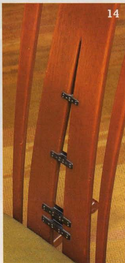
14. This chair's center splat appears to be pulling apart, but the ebony connectors secure the two halves in place. Gamble House living room rocker
