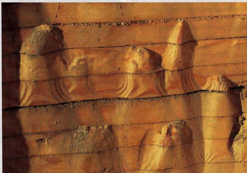
6 The abrasive, sandblasting action of grain flowing through the elevators over 100 years sculpted the interior edges of the planks. These surfaces are being saved for their unusual character.
