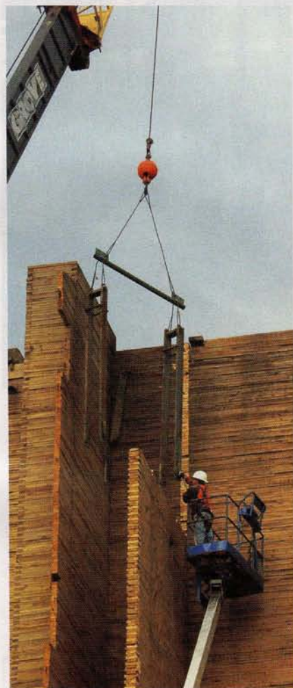
5 A pair of crane-suspended "tuning forks" are used to grasp segments of the elevator walls so they can be cut with chain saws and lowered to the ground.
