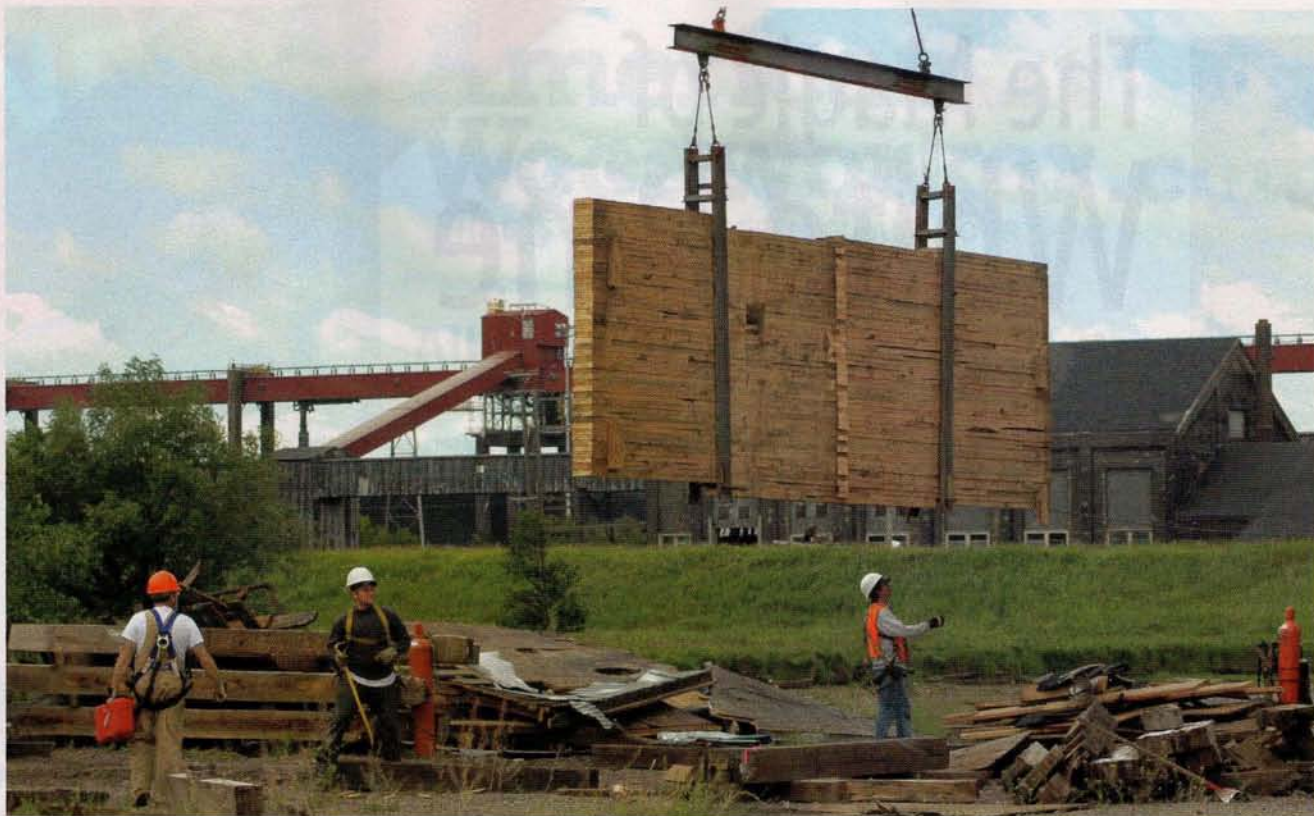
7 A small crew is working with a single crane to dismantle the three colossal elevators that made up the complex. The work is expected to take several years.
