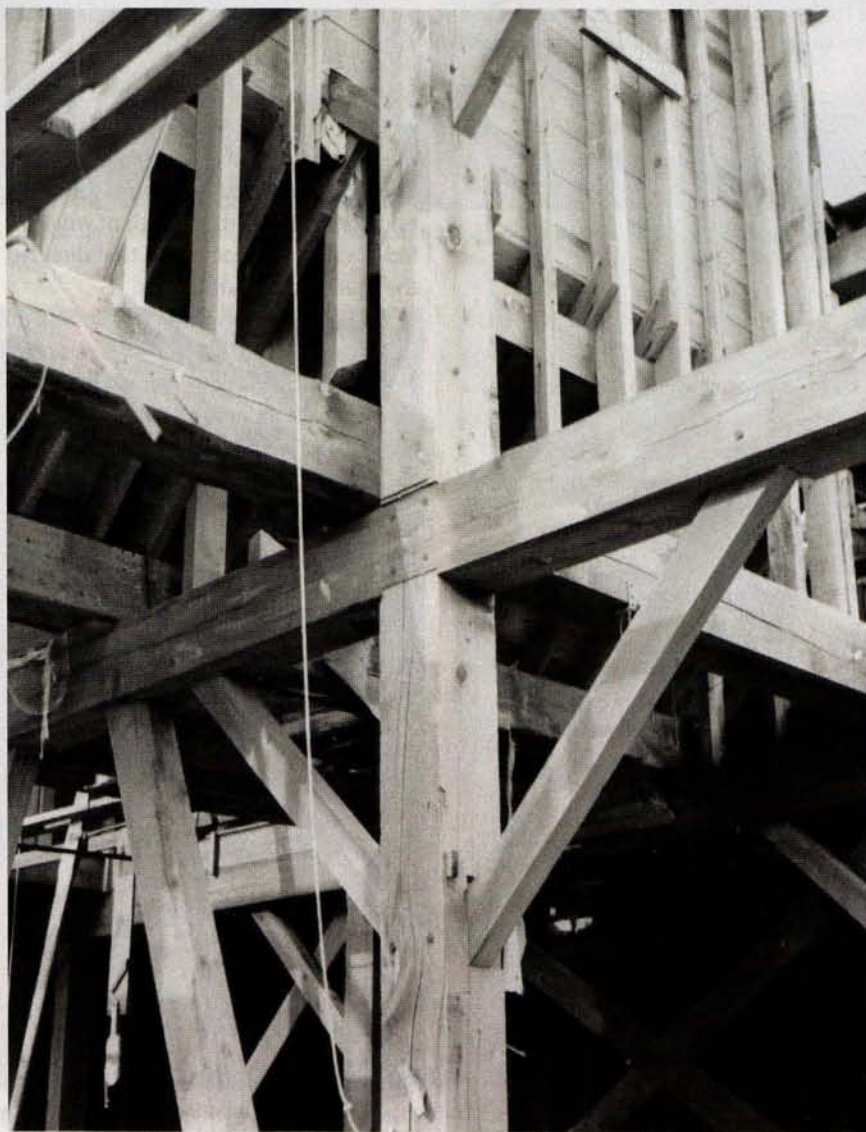
3 The ground and top floors of the elevator buildings were timber-framed with braced posts and beams.
