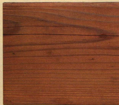
Finished with pigmented exterior oil, this section of the board looks virtually brand-new.
