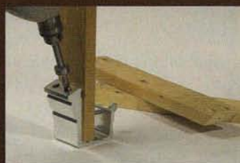
Drill into pre-aligned holes
