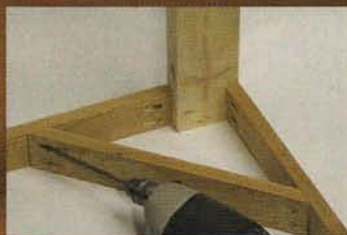
Assemble angle joints
