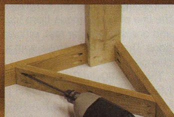
Assemble angle joints
