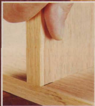
This blind dado joint is quick to make and nearly invisible.
