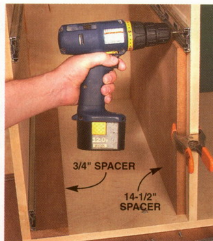
2 Spacer boards make it easy to install the drawer slides in the cabinet. The 3/4-in. spacer is also used to position the drawer members up from the bottom edge of the drawers.
