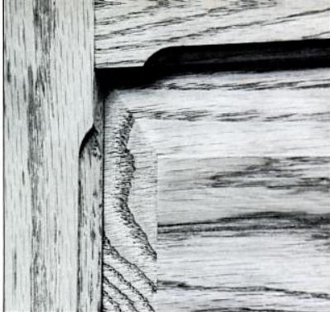
Ornament the rails and stiles surrounding the panels with a round-over profile.
