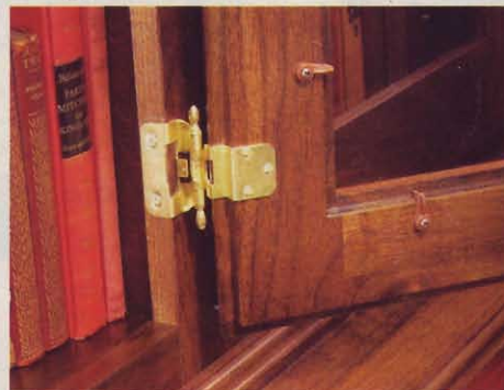
Lipped doors are easy to fit and hang and will even hide gaps caused by the doors being slightly warped or out of square.
