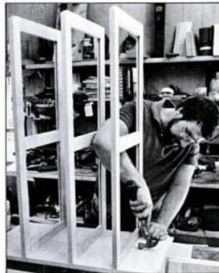
Glue and nail sides and frames together: Install the three center frames first. Glue and nail each joint with 1\frac{1}{4} -in. finishing nails at an angle, through the frame edges and into the sides of the dados.
