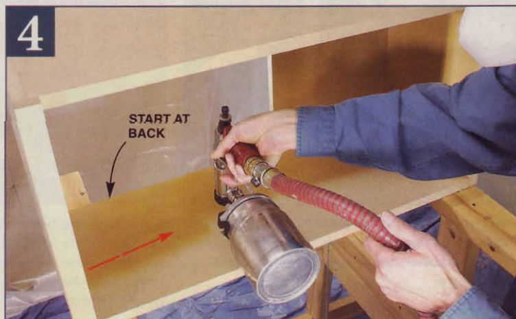
Spray the sides , moving from back to front, away from the overspray.
