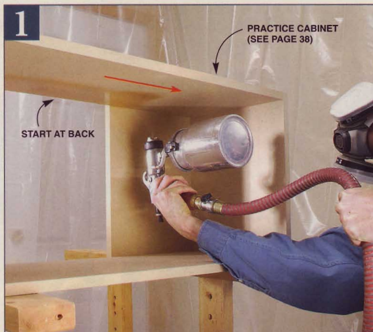
Spray under the top , moving from the back to the front. The fan pattern should just reach the edge of the cabinet back.
