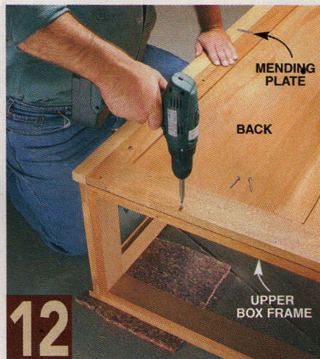
12 Screw the back to the top and bottom box frames. Add a mending plate along the side to hold the back to the side leg.
