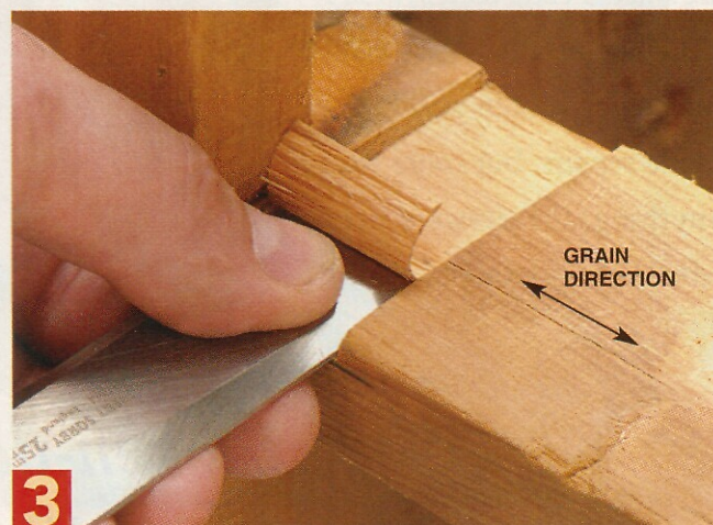
3 CHISEL OUT THE WASTE, to create a flat-bottomed dado. Then glue in a patch, with the grain direction of the patch the same as the divider.
