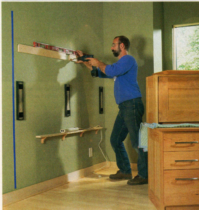
Photo 24 INSTALL THE CABINETS by laying out two strips of masking tape that are perfectly plumb. Then measure up from the floor and in from the tape to locate the hanging strips for the upper cabinets, the mounting boards for the bulletin board, and the narrow shelf that holds the power strips.
